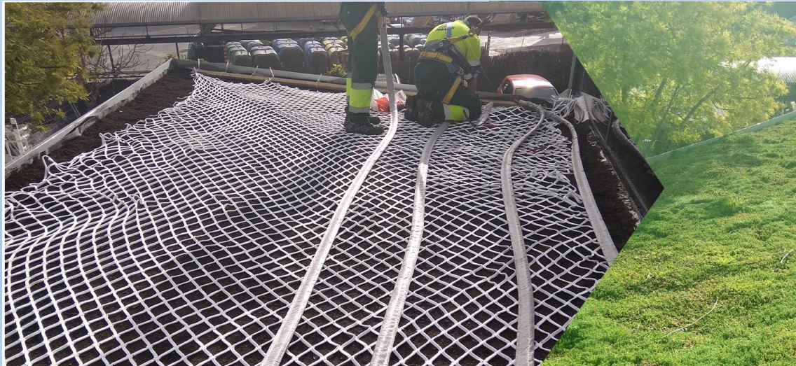
net-shaped textile with coated drip irrigation tubes (roof greening example) – system placed individually at root level
